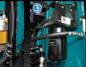
Pre-filter with integrated water separator
