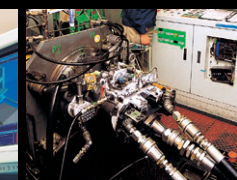
Main pump testing area
